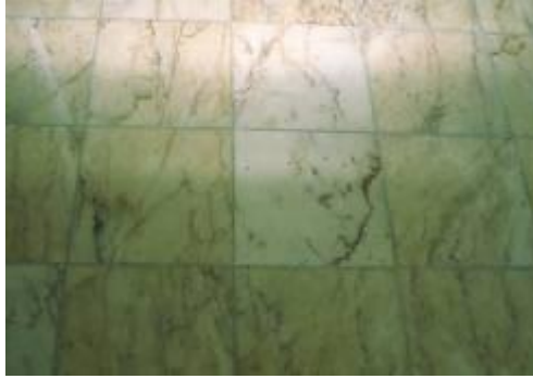
Figure 1: case of discolouration of a marble
